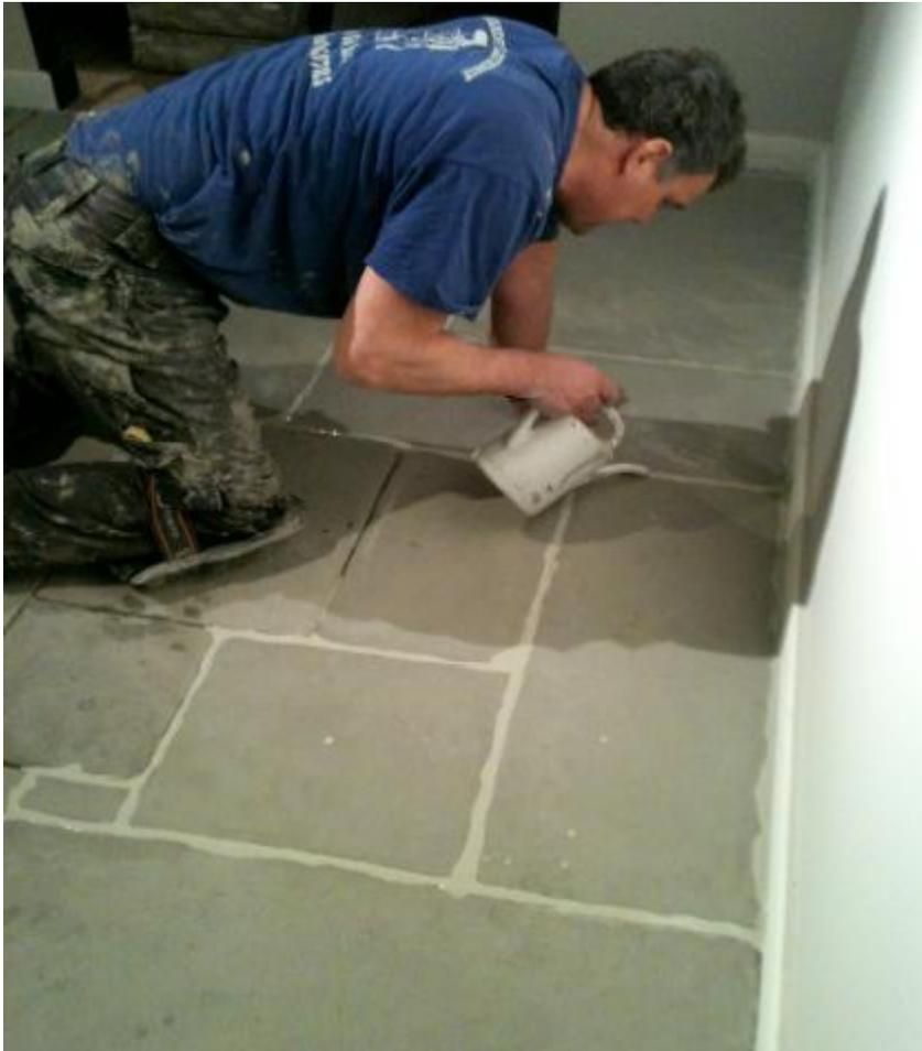
Using a large sponge and clean water dissolve the white haze and repeat this procedure after laying about 10 m<sup>2</sup>. Make sure the haze is dissolved completely. The tiles should be smooth now without a coarse sandy feeling.
